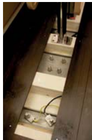
Keelbolts and backing plates are easily accessible
